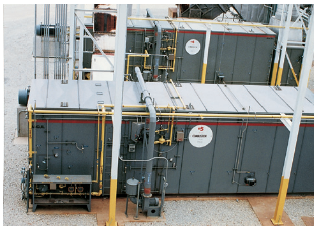
LEFT: VOC tailgas control for formaldehyde manufacturing plant.
